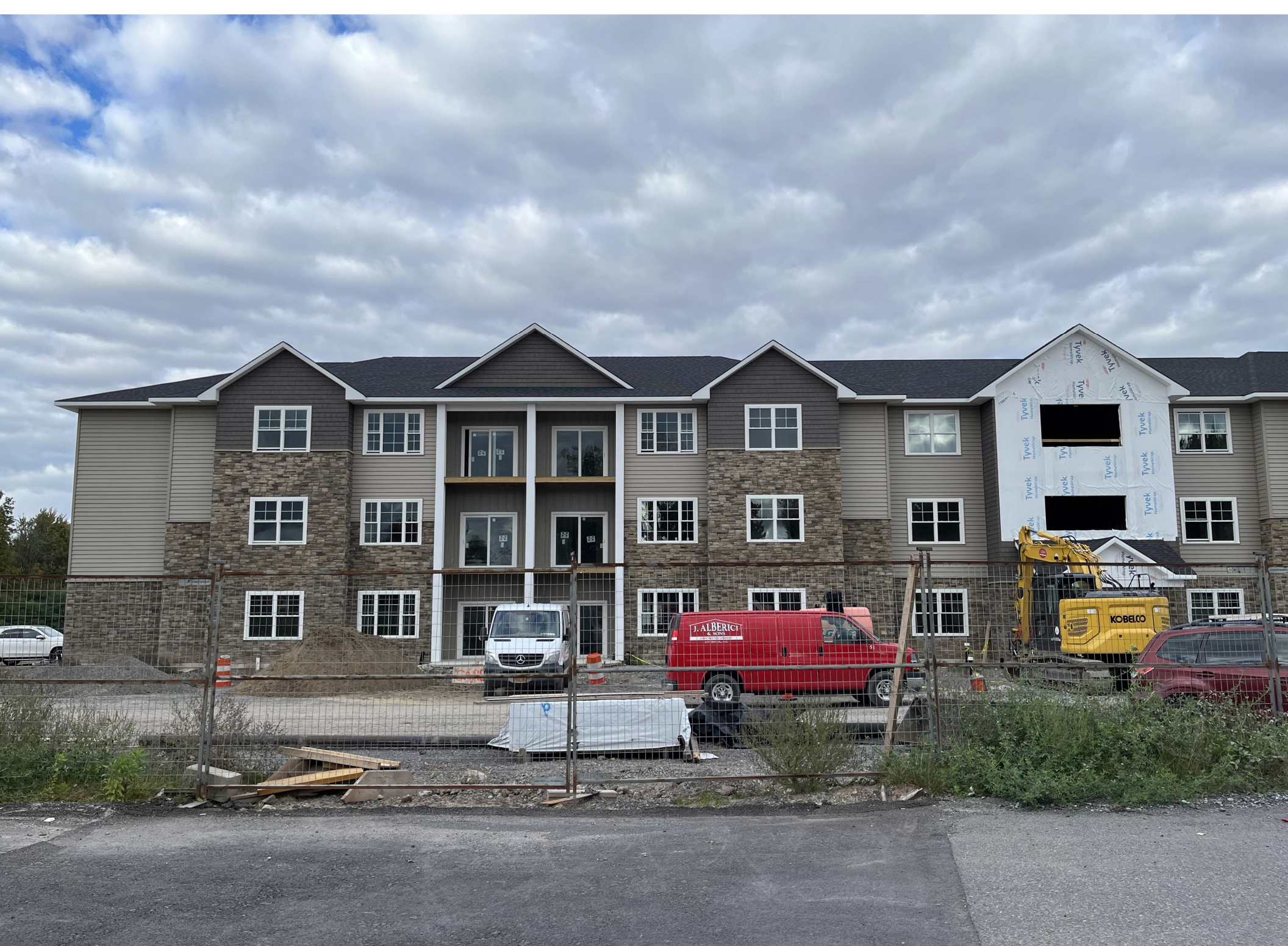
Treeline Apartments Under Construction - Color/Stone Example ( 7540 Buckley Road)
